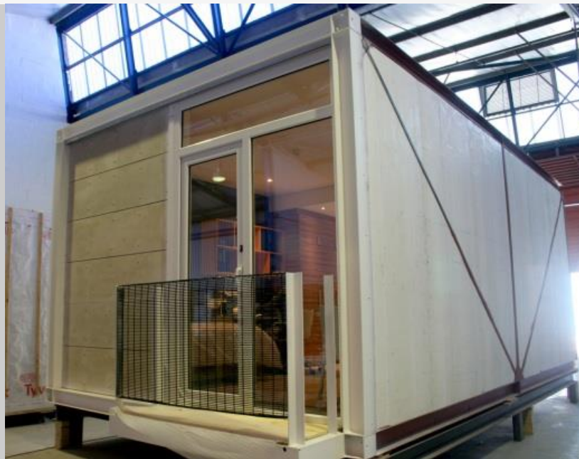
Factory prototype – note vierendeel frame on short elevation and bracing along the side.
